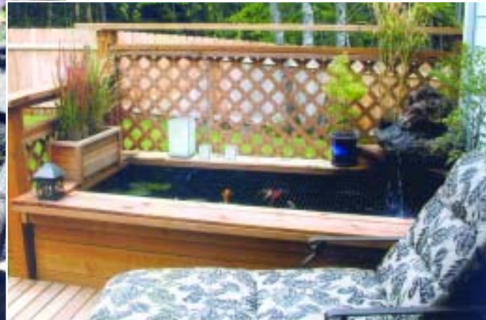
Fenix Theuerkorn of Bainbridge Island designed and built their 4 x 8' pond to be 3 feet deep for their 8 young koi. The readily accessible deckside pond is serviced by a Cyprio Bioforce 1000 pump and UV.
