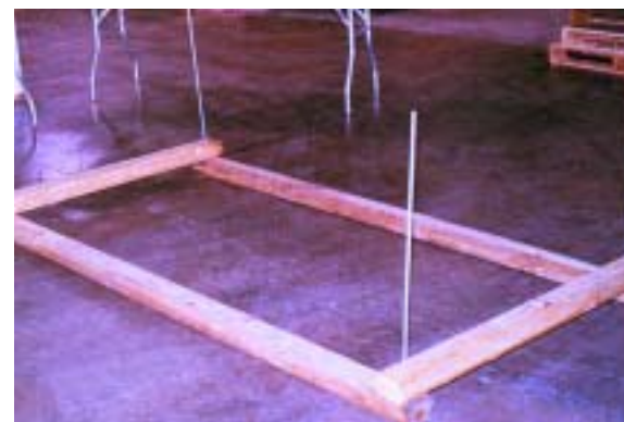
1. To build a landscape timber pond, cut some 8-foot-long timbers in half to form a 4x8-foot frame. Drill holes a couple inches in from each end so that the timbers can be anchored on a long post screw.
