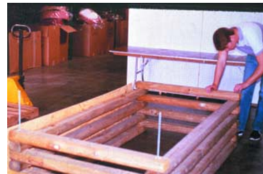
3. Build your timber walls as high as desired.
