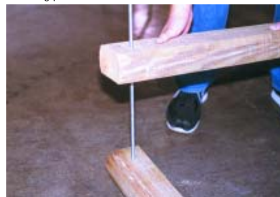
2. Add timbers alternating from length to width sections as though you were building a log cabin.
