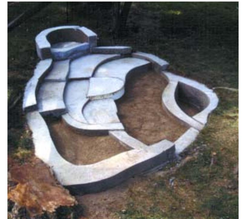
Concrete was mixed by the bag and filled into each section of the forms. The 12-inch railroad spikes holding the forms in place were pulled before the concrete had fully set.
