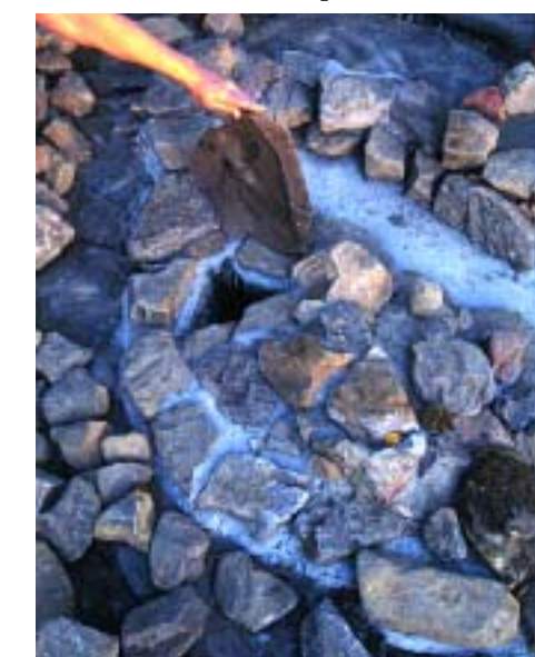
(bottom) The reservoir is camouflaged with stone over and around a plastic-coated grate. The capstone is left free of mortar for easy access to the submersible pump.
