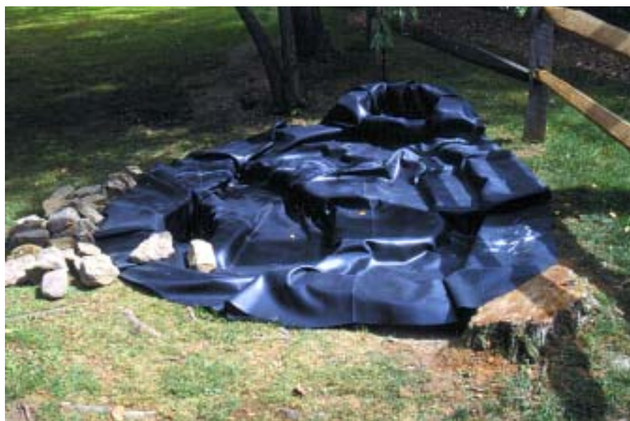
Fully lining the entire construction prevents water loss.
