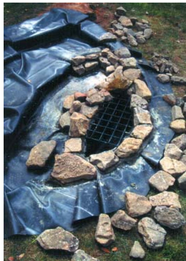
(above) Because the shallow bird pond covers about 80 square feet, a 50-gallon, hidden reservoir will provide the water source.
