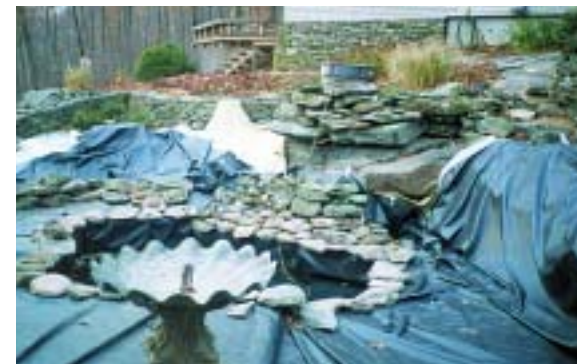
The pond excavation is fully lined.
