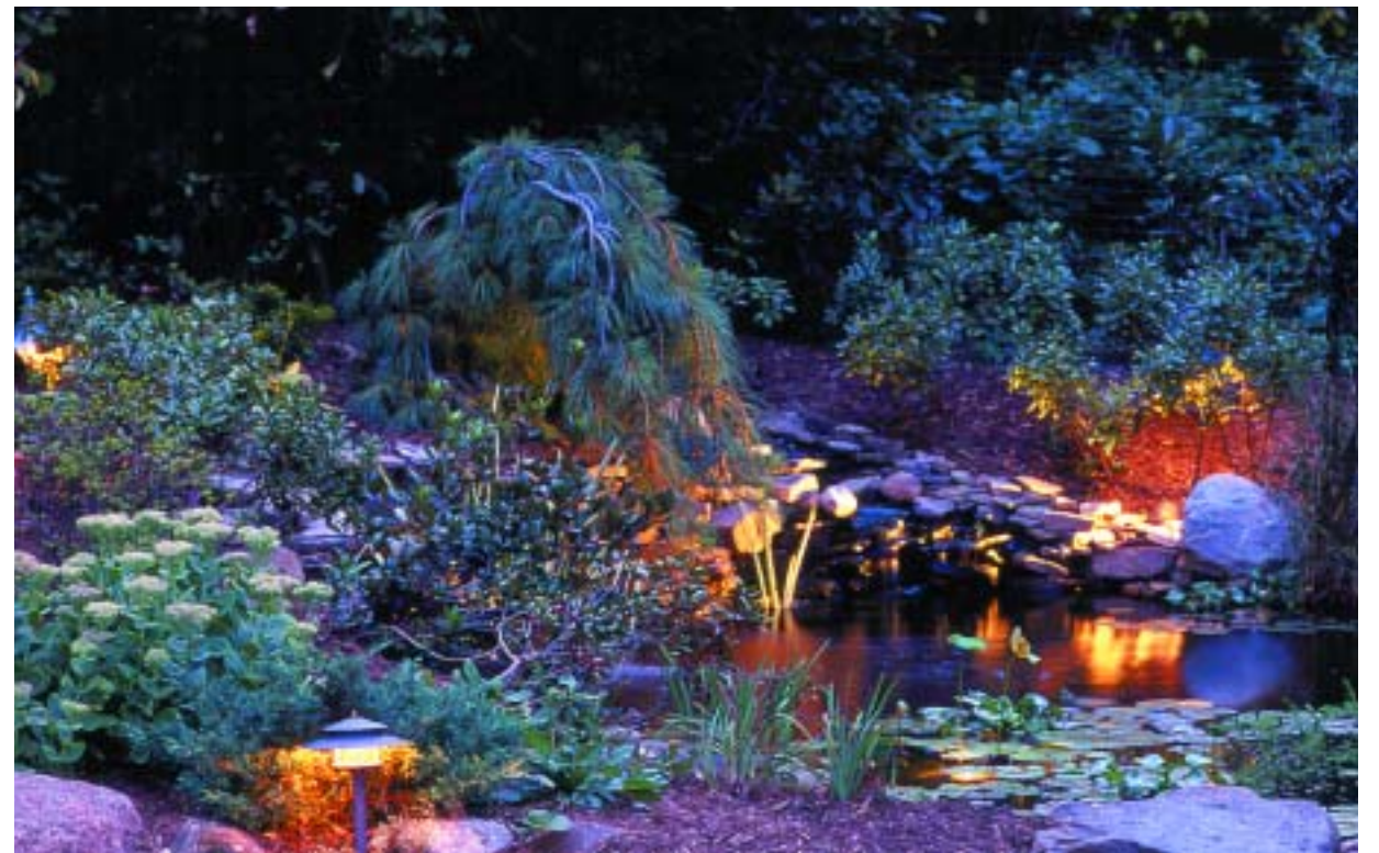
Lights surrounding this pond include various pathlights used to highlight plantings, a light in the pond, which will silhouette the water lilies after total darkness, and the hidden spotlight shining across the waterfall.
