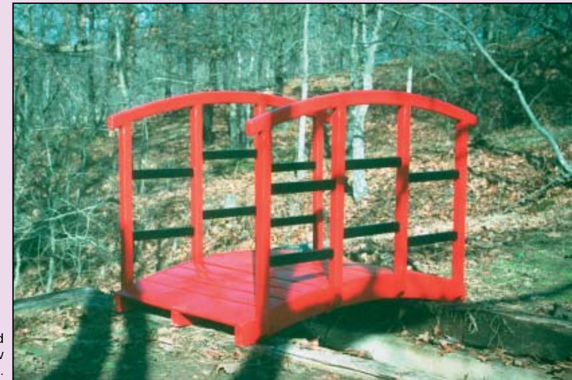
The completed bridge over narrow dry stream bed.
