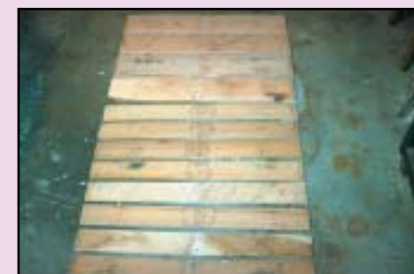
Closeup showing floor connections
