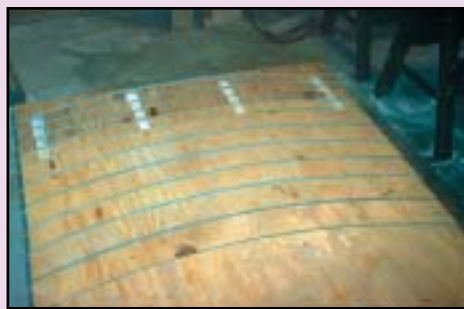
Floor panels laid out from pallets
